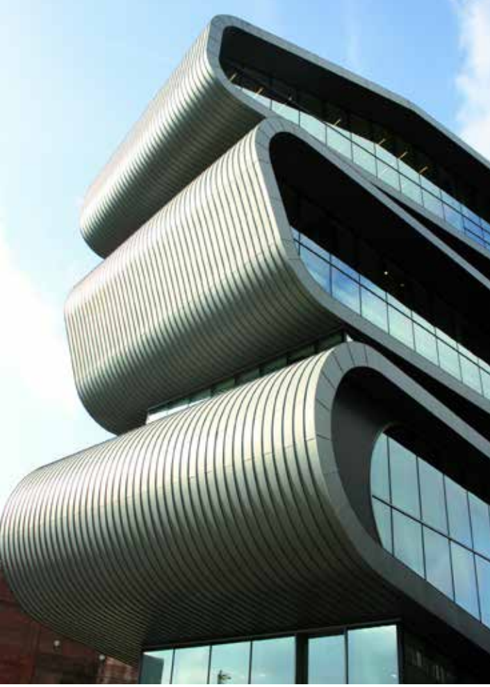
VMZ Dik kenet tonoz kabuk cephe, QUARTZ-ZINC®
